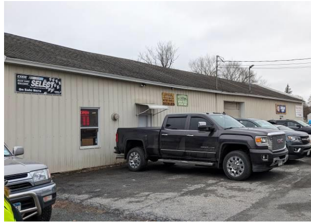
Photo No. 4 North side of 1842 NY-67 looking west along NY-67.
