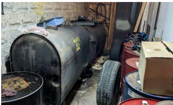
Photo No. 11 Two (2) used oil ASTs stored along the northern wall of the southern storage area.
