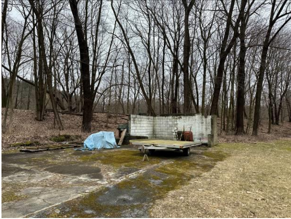
Photo No. 13 50 State Street demolished portion of the former NYSDOT building.
