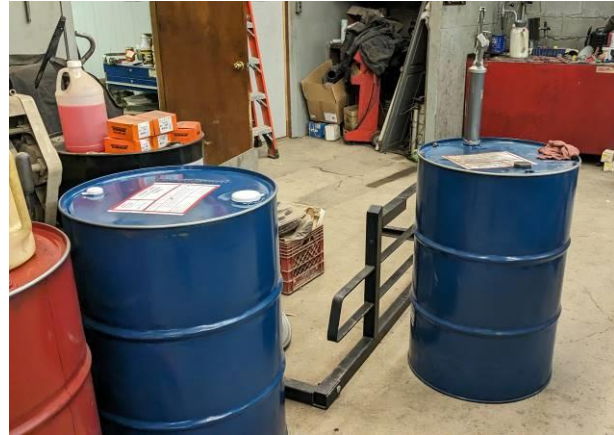
Photo No. 8 New coolant and oil 55-gallon drums and new oil AST located on the eastern portion of the garage bay.
