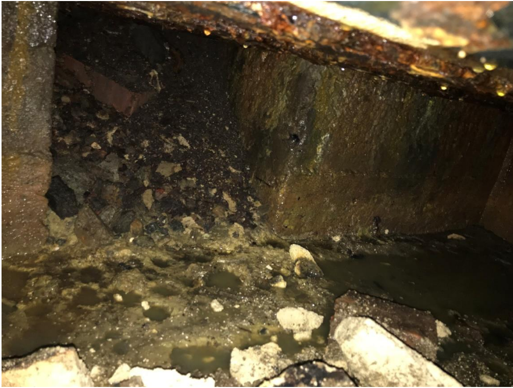
3.) Test Pit 1: Looking North towards river. Depth of chamber approx. 1 foot.
