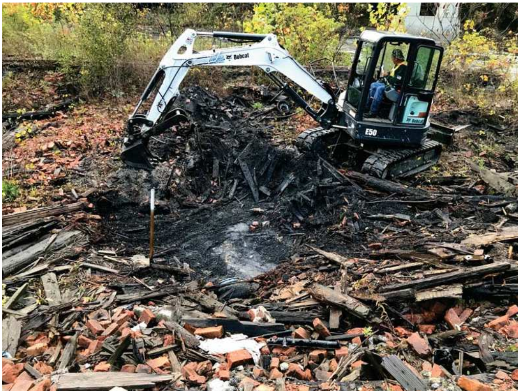
Photograph 3: TP 2, View to North
