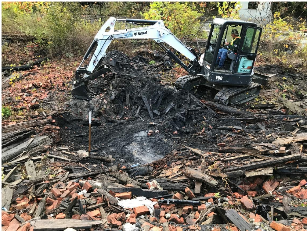
4.) Test Pit 2: Looking North towards river. Concrete slab located approx. 1 foot below top of rubble. Excavation ended here.
