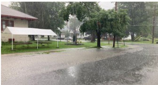
Poor stormwater drainage along State Street impacts the Valley Falls Free Library.
