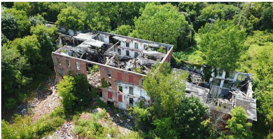
Existing condition of the Thompson Mill property
