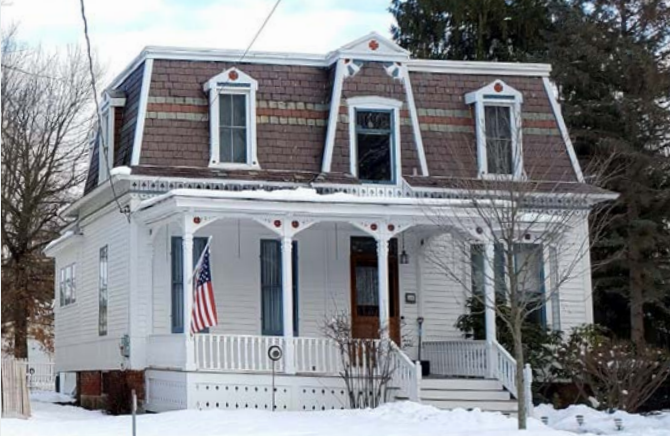
Mansard Roof at 26 State Street
