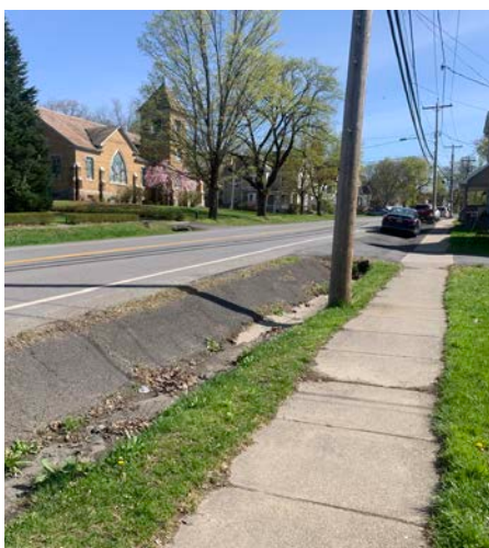
Existing condition of the open drainage along State Street
