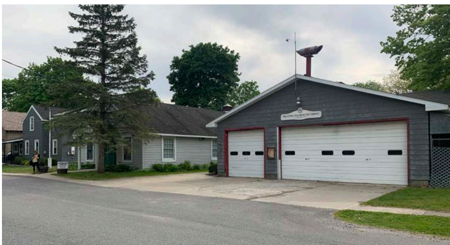
Existing condition of the Village Hall and former Fire Department
