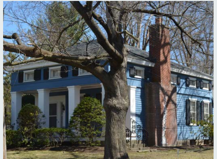
Greek Revival Features at 115 Bunker Hill Road Photo by Jessie A. Ravage, 2017
