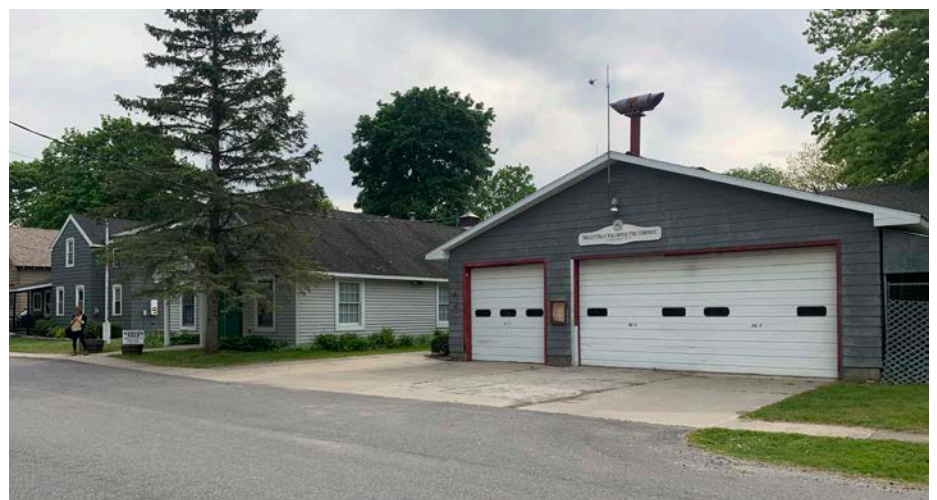
Existing condition of the Village Hall and former Fire Department
